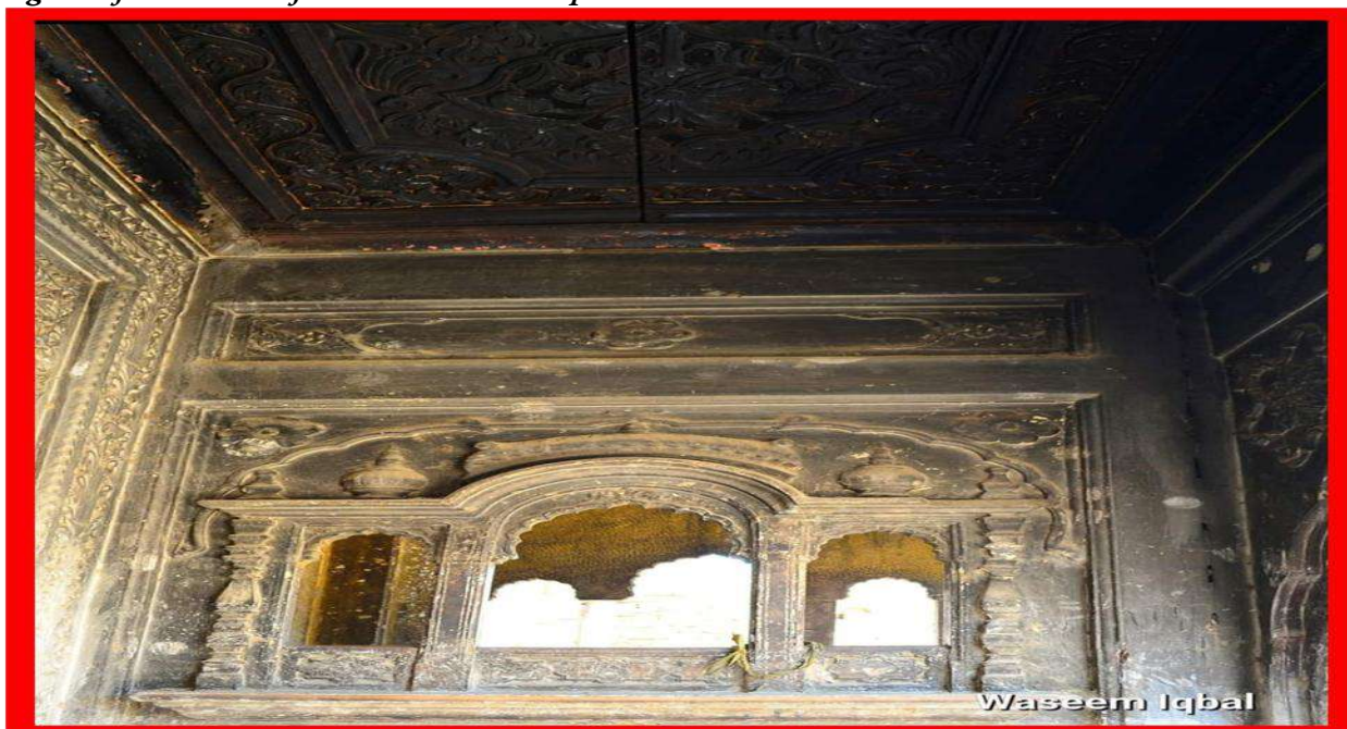
Fig.7. The Most sacred place of the Temple, visitors love flair the lamp with oil for Goodness of their Gods. Over the centuries this cabin of Lamp had been totally black out due the black dust of the burning lamp. The Roof of the Cabin much decorated with Wood work & side by side walls.
